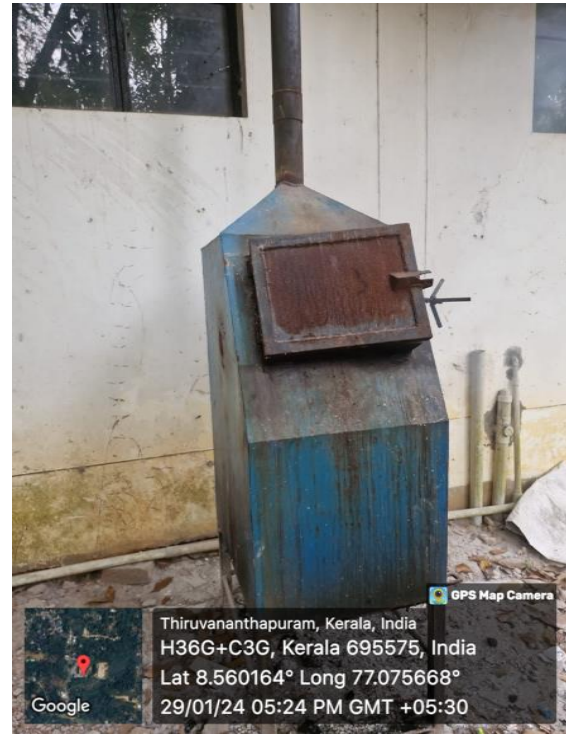
Outside section of incinerator
