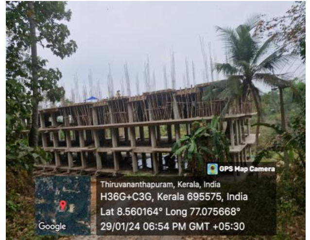
Hostel Facility (work in progress)
